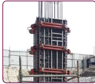
COLUMN FORMWORK
