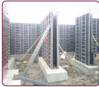
WALL FORMWORK
