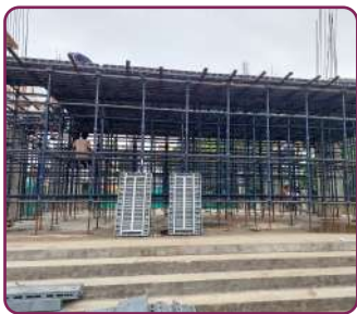
SLAB FORMWORK
