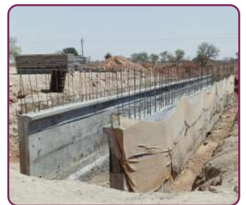
DRAIN FORMWORK
