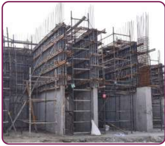
WALL FORMWORK
