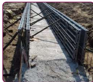
DRAIN FORMWORK
